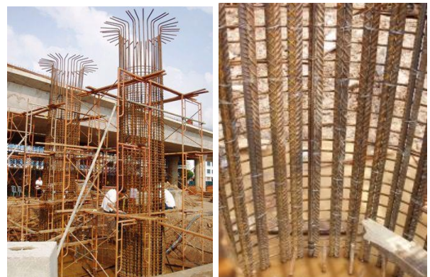
Road Bridge Pier monitoring, Malaysia
