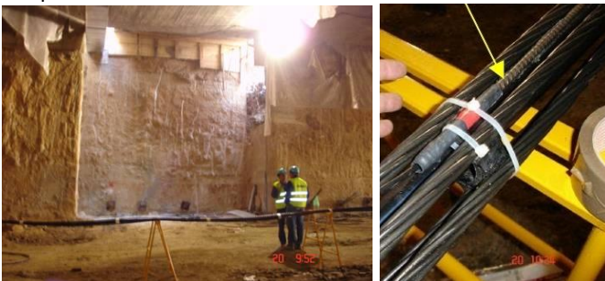
Diaphragm wall ground anchor tension, Spain
