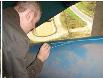
Road Bridge Superstructure
